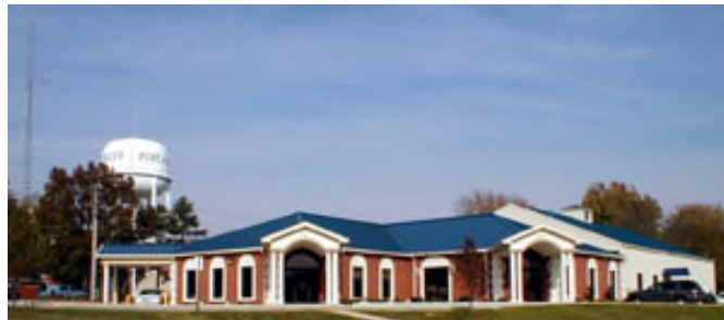
System Operations & Headend Building
